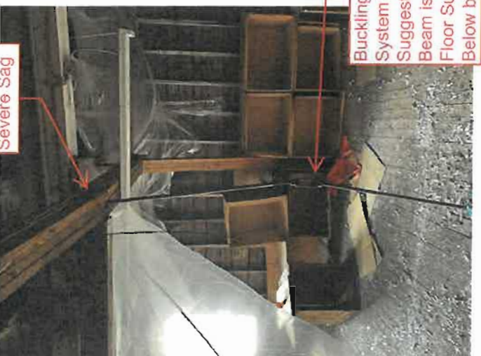
Second Floor/Roof Framing Support System Failing
