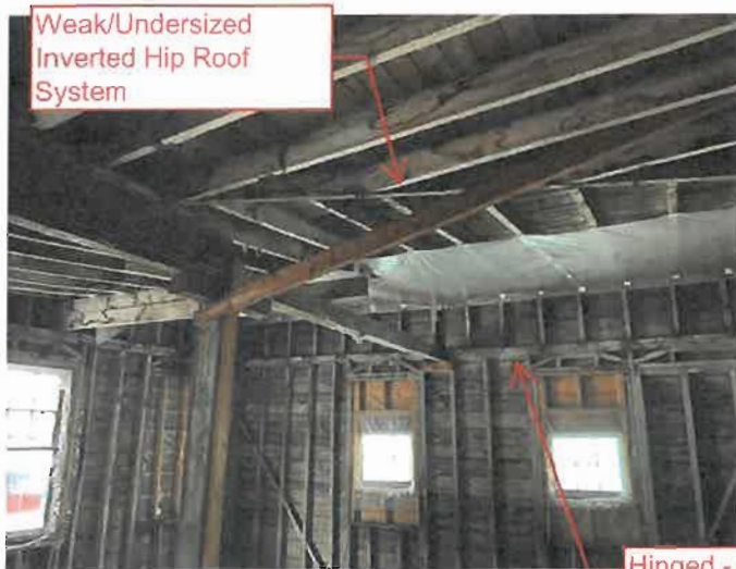
Hinged - Structurally Un-Sound 2nd Floor Walls All Around.
