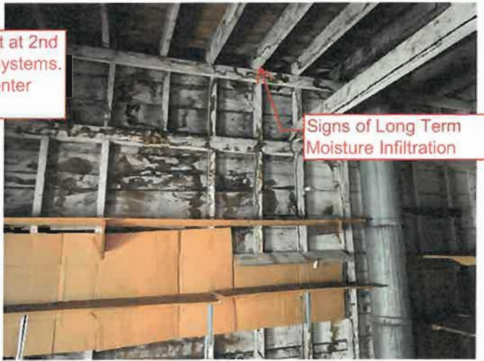
Roof Joist System Undersized
