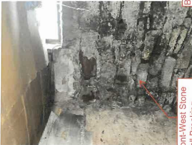
Back-East Wall not Straight and True
