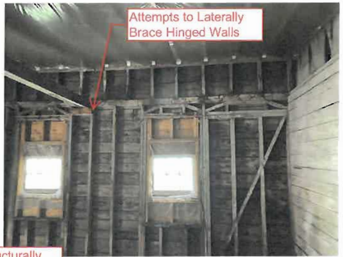
Hinged - Structurally Un-Sound 2nd Floor Walls All Around.
