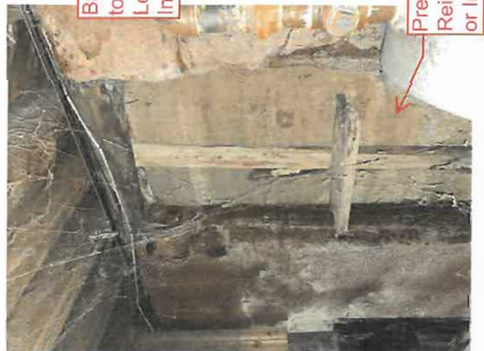
Brick Wall Starting to Break Down and Leaking/ water Infiltration
