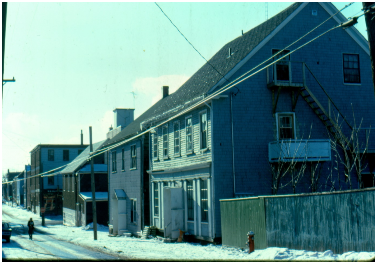
93 King Street & 91 King Street from east side
